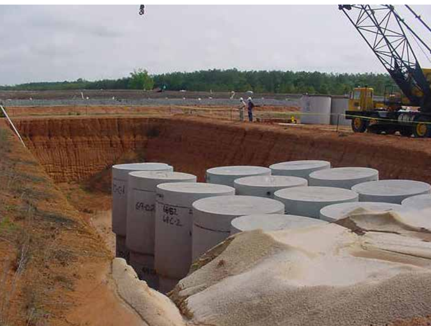
Regulating waste disposal is essential to making mining operations more sustainable.
